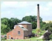
Completed in 1810, the beam engines are fed by water from springs close to Crofton Lock and topped up by Wilton Water, a reservoir created for the pumping station. Water
