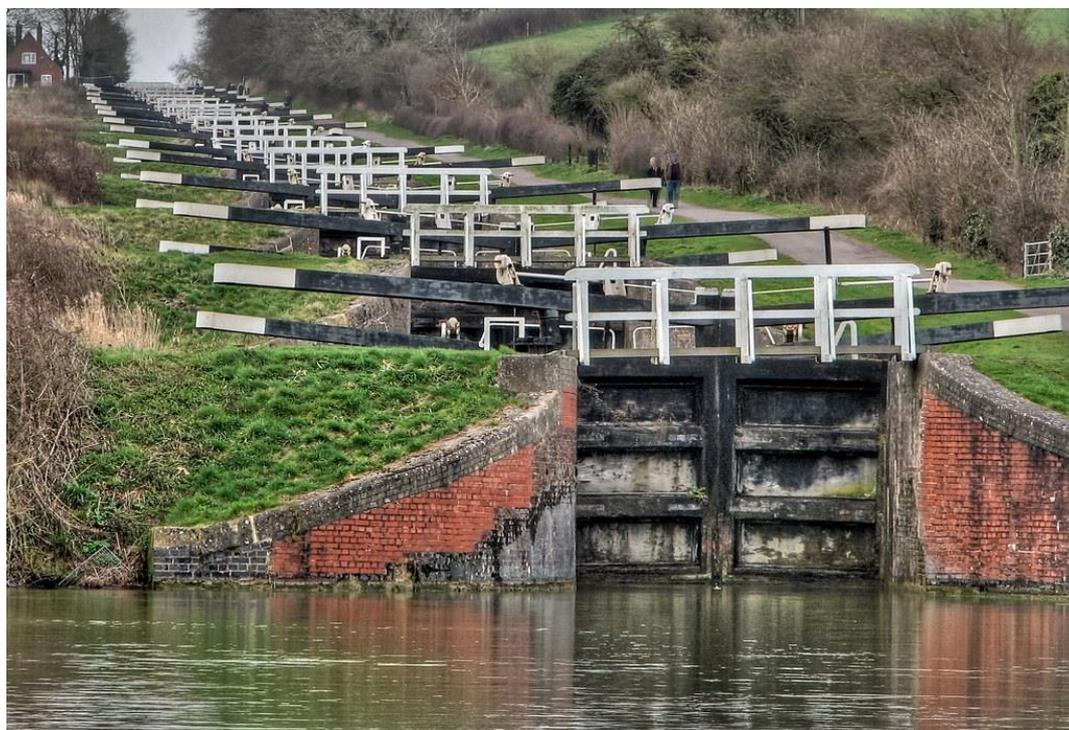
Completed in 1810 under the supervision of John Rennie the Elder, the Caen Hill Locks represent another remarkable feat of engineering in the building of the canal. A brick-making factory was built to provide the large number of bricks required to line the chambers of the locks. During the construction phase a horse-drawn tramway ran parallel to the canal route to convey goods across this stretch. Rennie had originally planned that the canal should be routed through Marlborough
